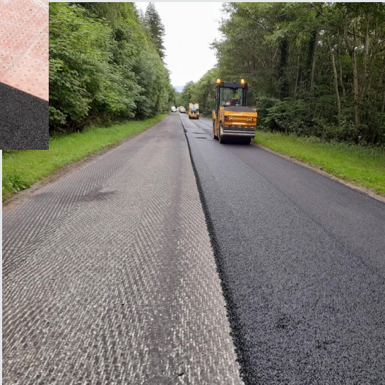
A835 carriageway resurfacing
