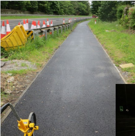
A702 Nine Mile Burn footpath construction
