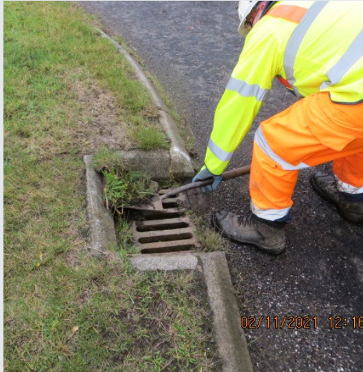
A68 North of Pathead gully and manhole cleansing
