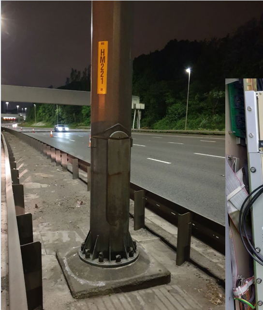
M8 high mast lighting cyclic maintenance
