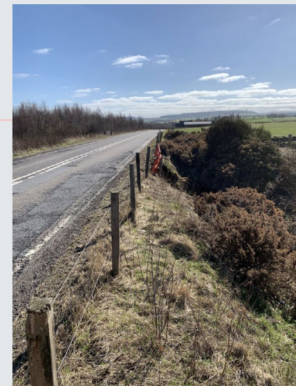
Proximity of failure to A96
