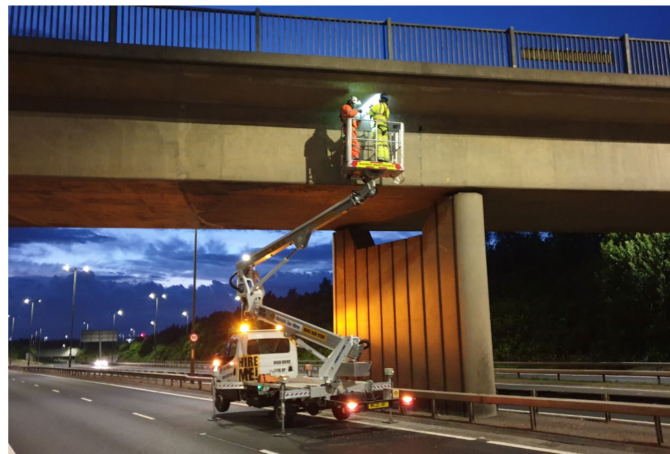
A720 Aqueduct – Post Tensioning system investigation
