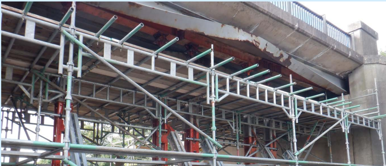
Temporary works and propping for beam replacement
