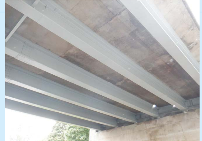
View of repaired beams from A90 carriageway level
