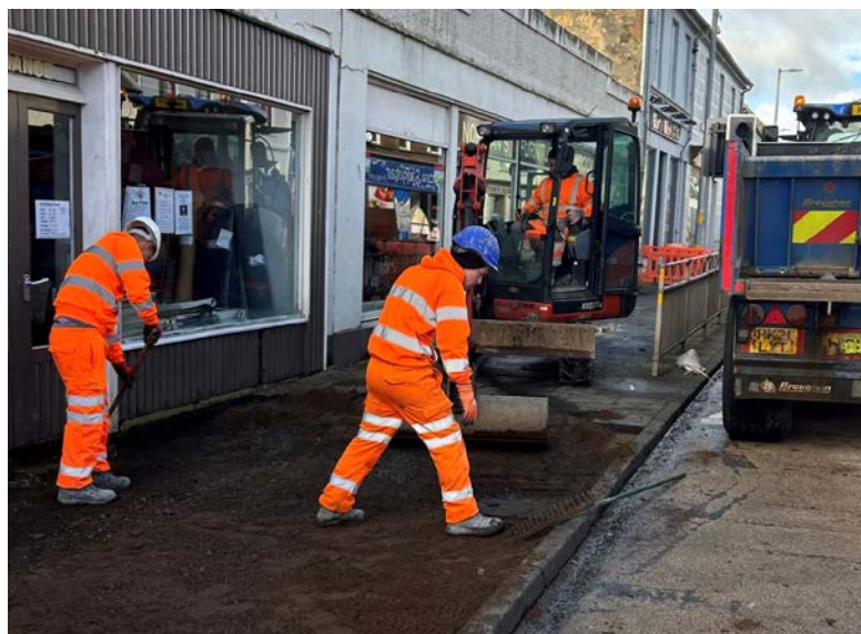
SW NMC: A75 footway resurfacing
