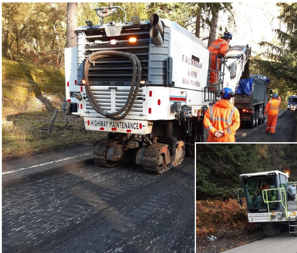
Figure 4 A86 Planing Operation
