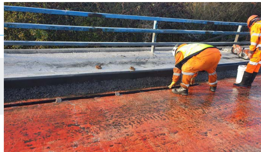
SW NMC: M74 Bridge refurbishment
