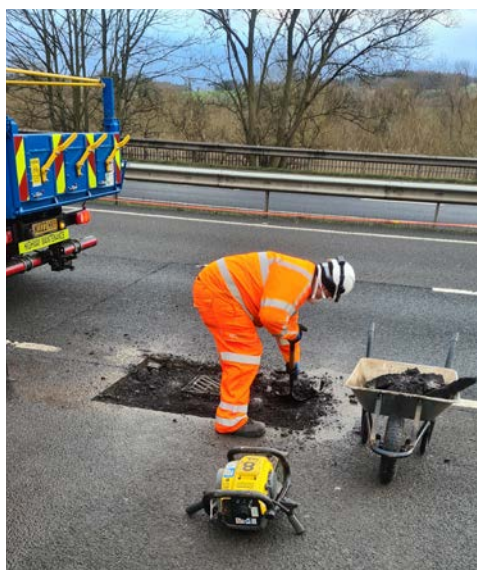
NE NMC: A90 Category 1 Repair
