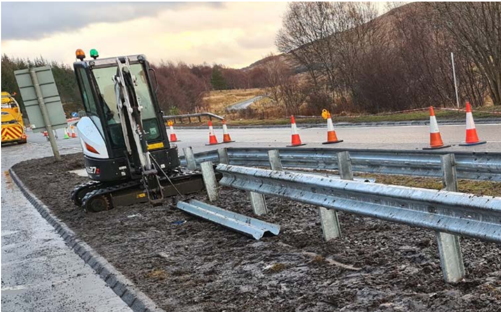
NW NMC: A9 Vehicle Restraint System replacement
